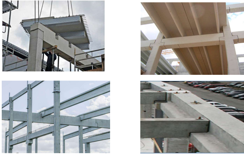
Figure 1. Some joints configurations in two crossed precast beams.
