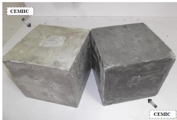
Figure 8. Visual inspection of CEMIC and CEMIIIC 150 mm cubes after 365 days
